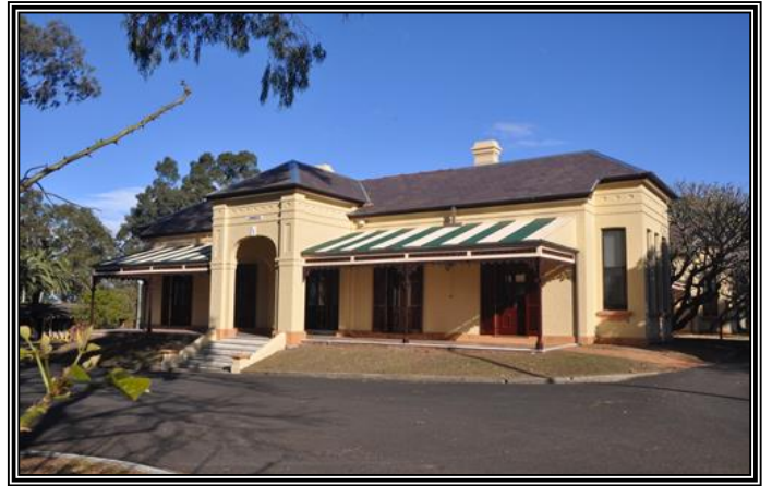
Linnwood – Listed on the NSW State Heritage Register
